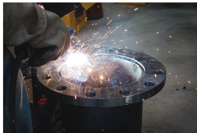
Overlay of pipe flange Supercored 309MoL
